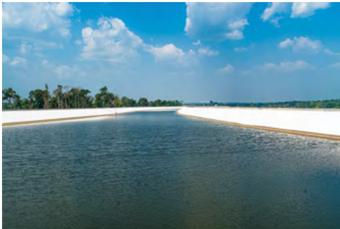
Water flows from the conduit canal of the retention dam to the water intake dam
